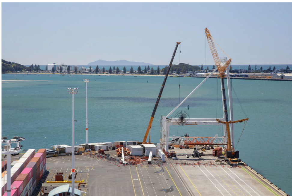
Figure 1: assembly of a new crane at Sulphur Point
